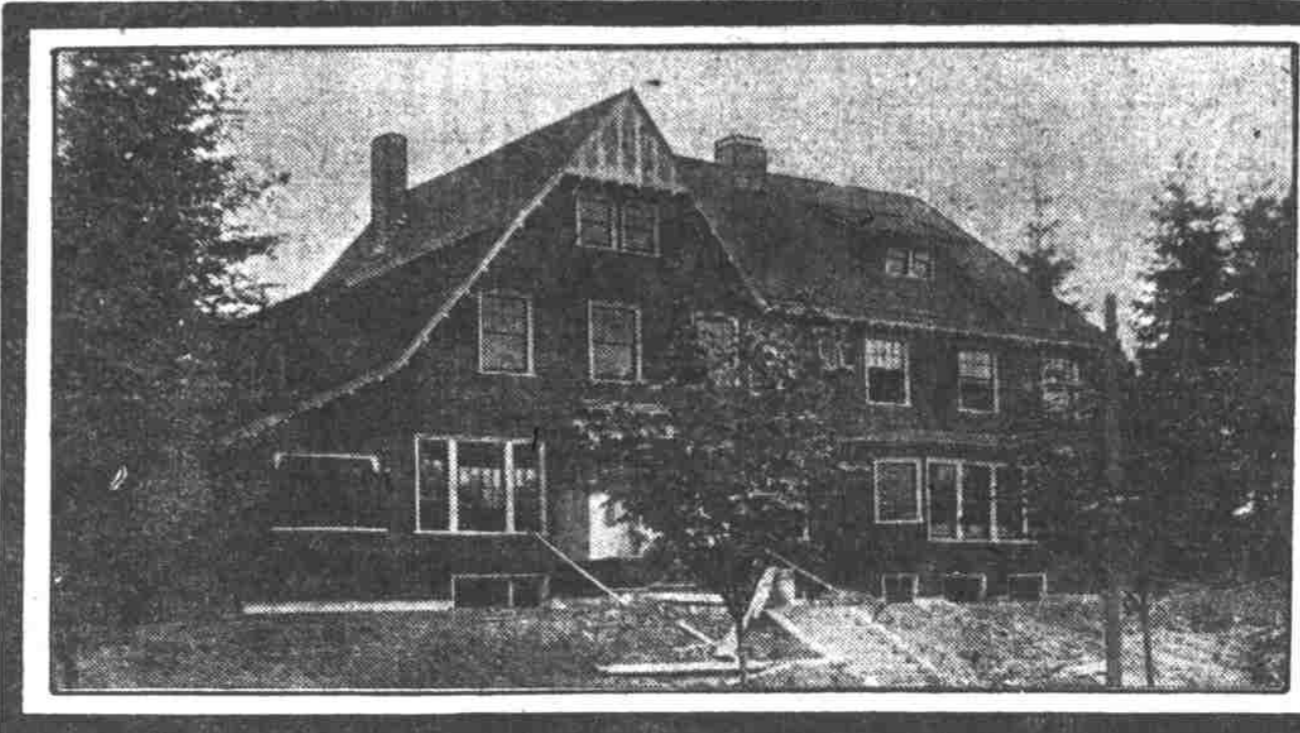
RESIDENCE OF E. F. LAWRENCE, E. 21ST & TILLAMOOK.
