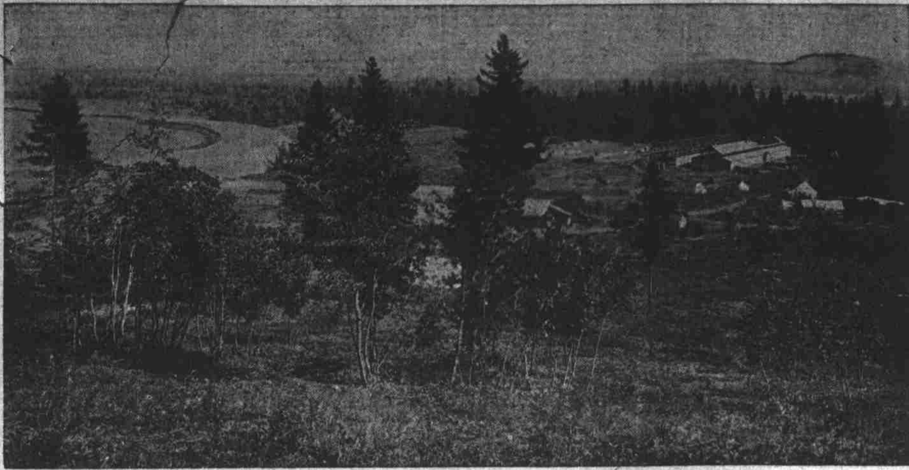
West End of Country Club's Grounds, Showing Work So Far Completed on Exhibit Barns.
