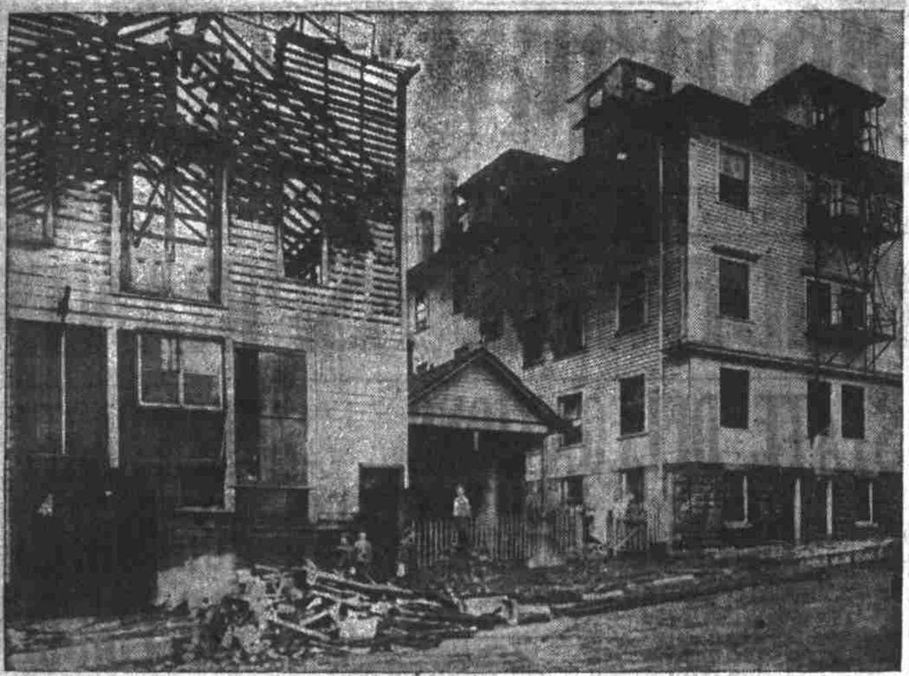
Westminister apartments damaged in early morning fire.
