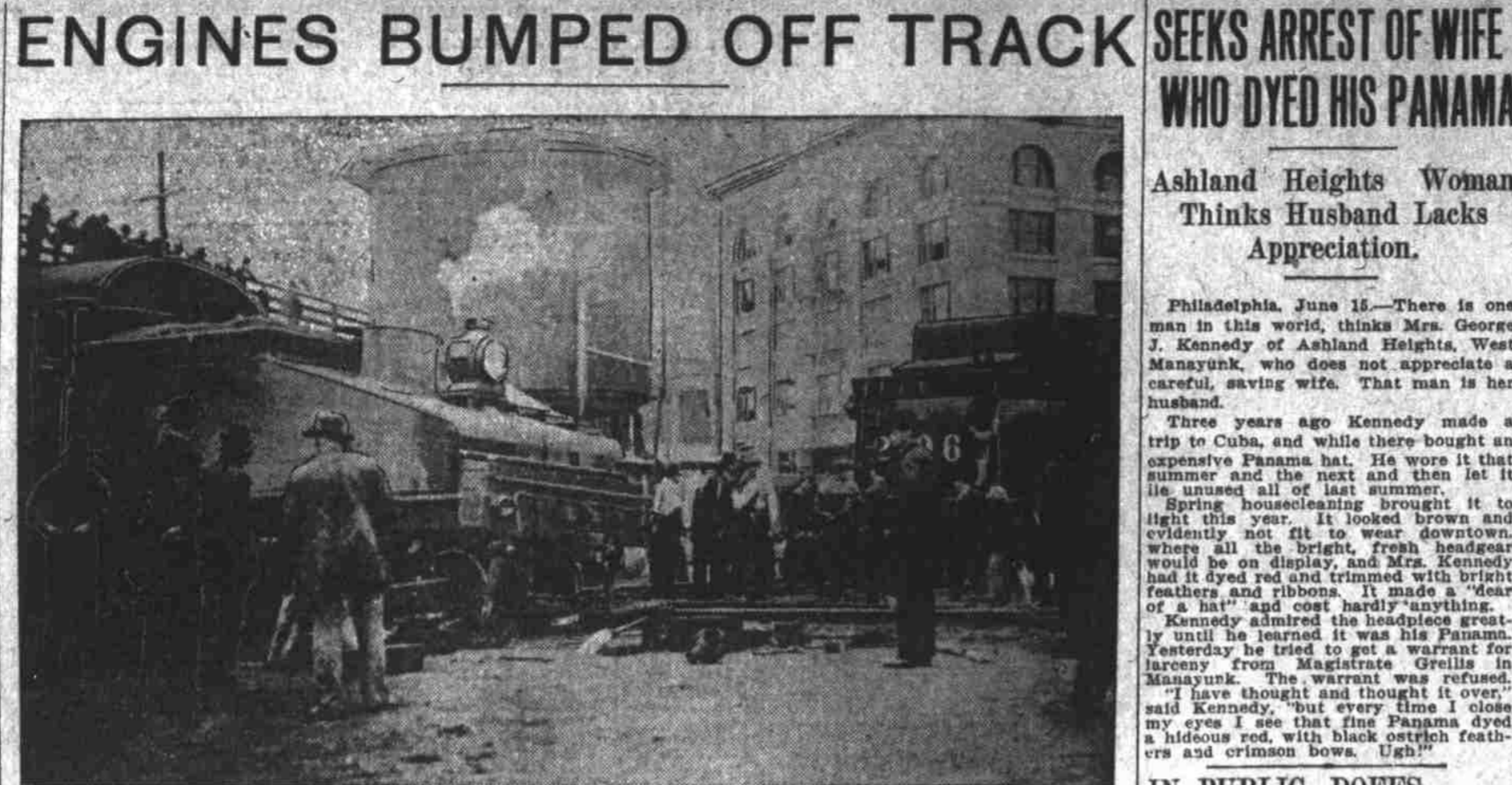
Putting the bucking locomotives back on the track.
