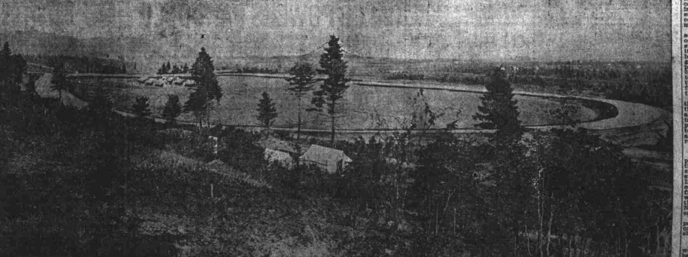
Mile Race Course Under Construction on the Grounds of the Portland Country Club and Livestock Association.
