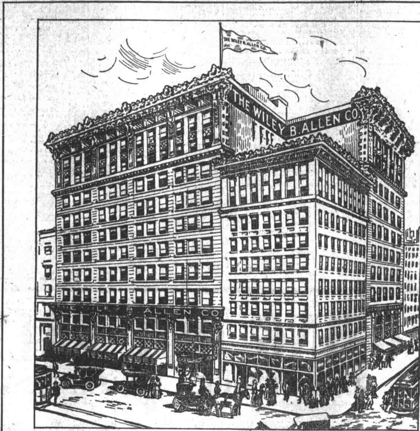
The new headquarters of the Wiley B. Allen Company, now under way of construction at the corner of Kearny and Sutter streets, San Francisco. One of the largest establishments in the world devoted exclusively to the sale of pianos.
