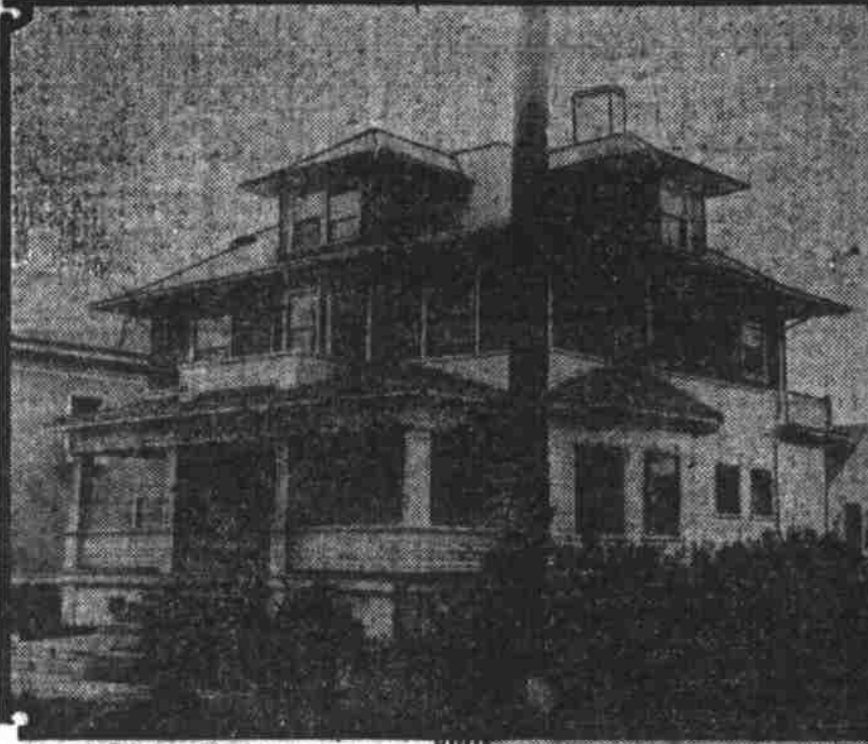
RESIDENCE OF H. B. STOUT 23RD AND RALEIGH ST.
