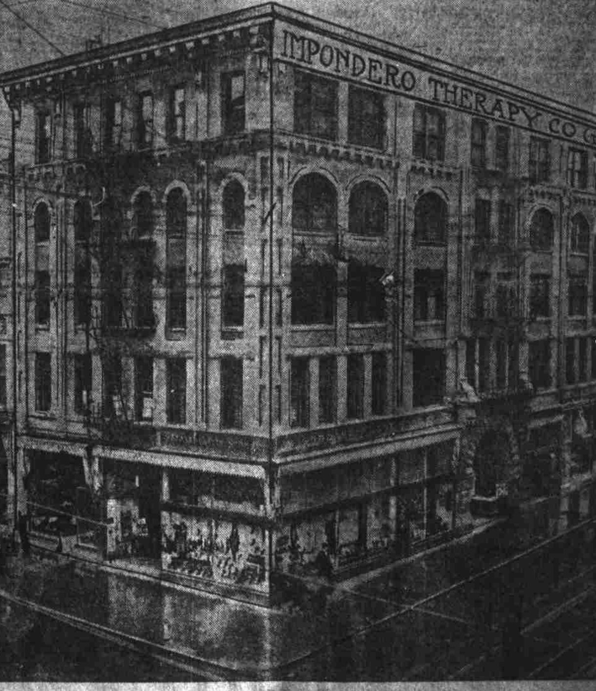
New home of the Impondero Therapy Company in the Merchants' Trust Building, 326 1/2 Washington Street, corner of Sixth.
