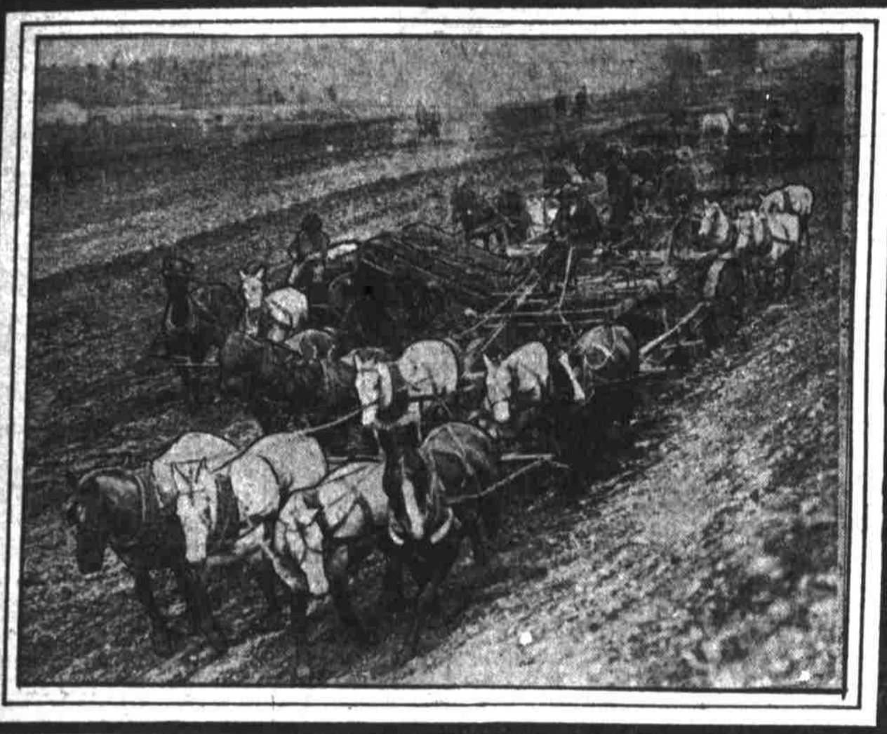
Mr. C. Connelly, foreman of the graders at Rose City Park, has invented a scraper that beats anything that has been tried in Portland for removing dirt and leveling lots. The scraper works in such a manner as to require no shoveling by hand after the scraping work is done. The dirt is carried by an endless chain into a wagon that drives alongside the machine. Mr. Connelly is justly proud of his invention.
