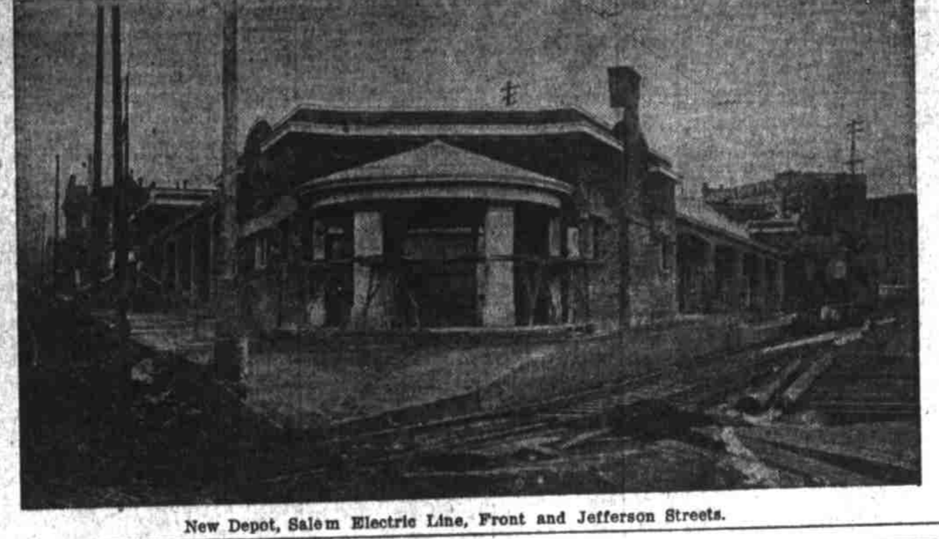
New Depot, Salem Electric Line, Front and Jefferson Streets.
