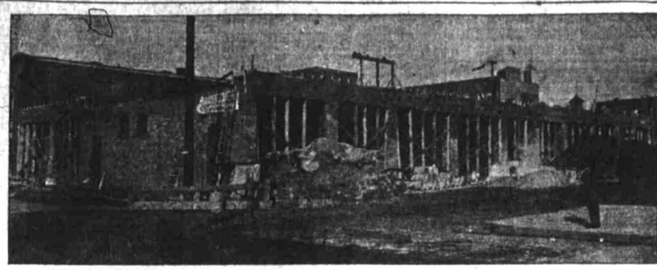
Dammer Building, Under Construction, at Fourth and Everett Streets.
