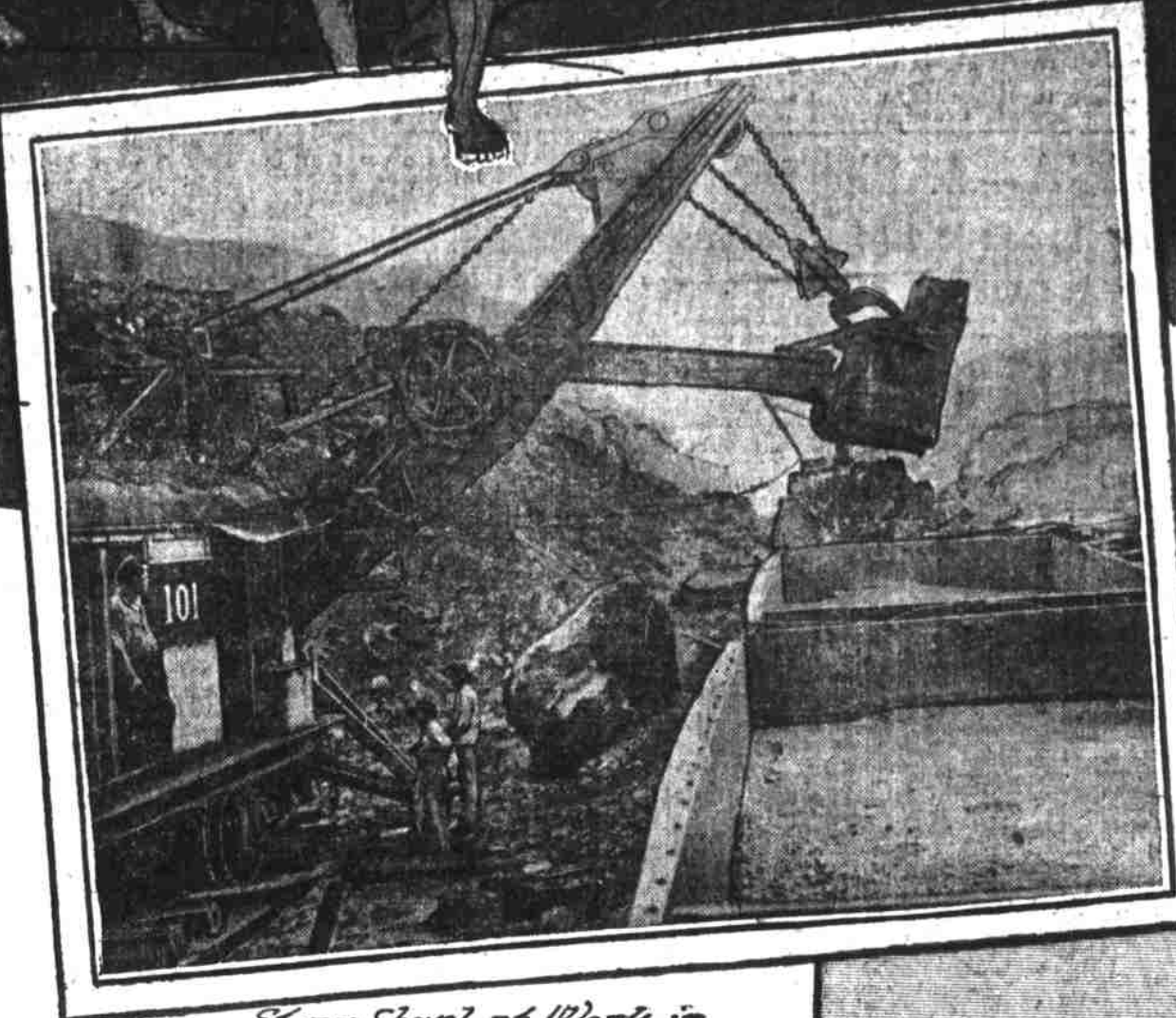
Steam Shovel at Work in Culebra Cut.
