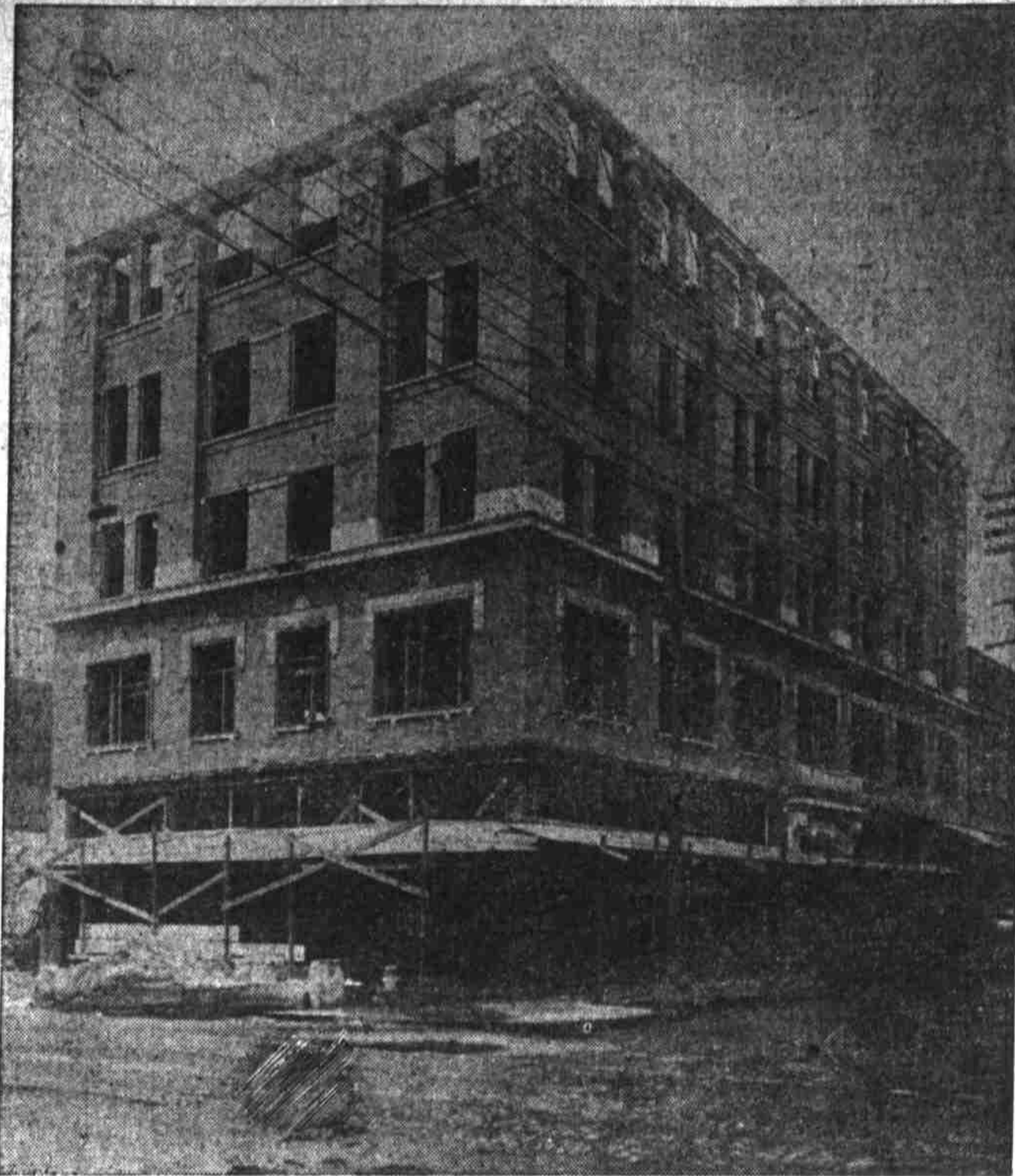
Gerlinger Office Building, Second and Alder Streets.
