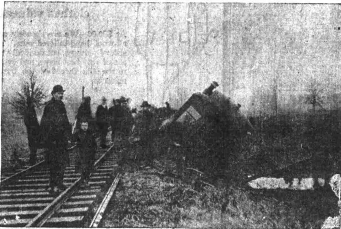
The photograph shows the rear end of a passenger coach of the wrecked train. A wrecking crew is today trying to raise the coach with lifting jacks.
