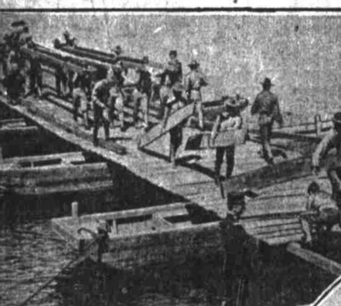
West Pointers Laying Pontoon Bridge.
