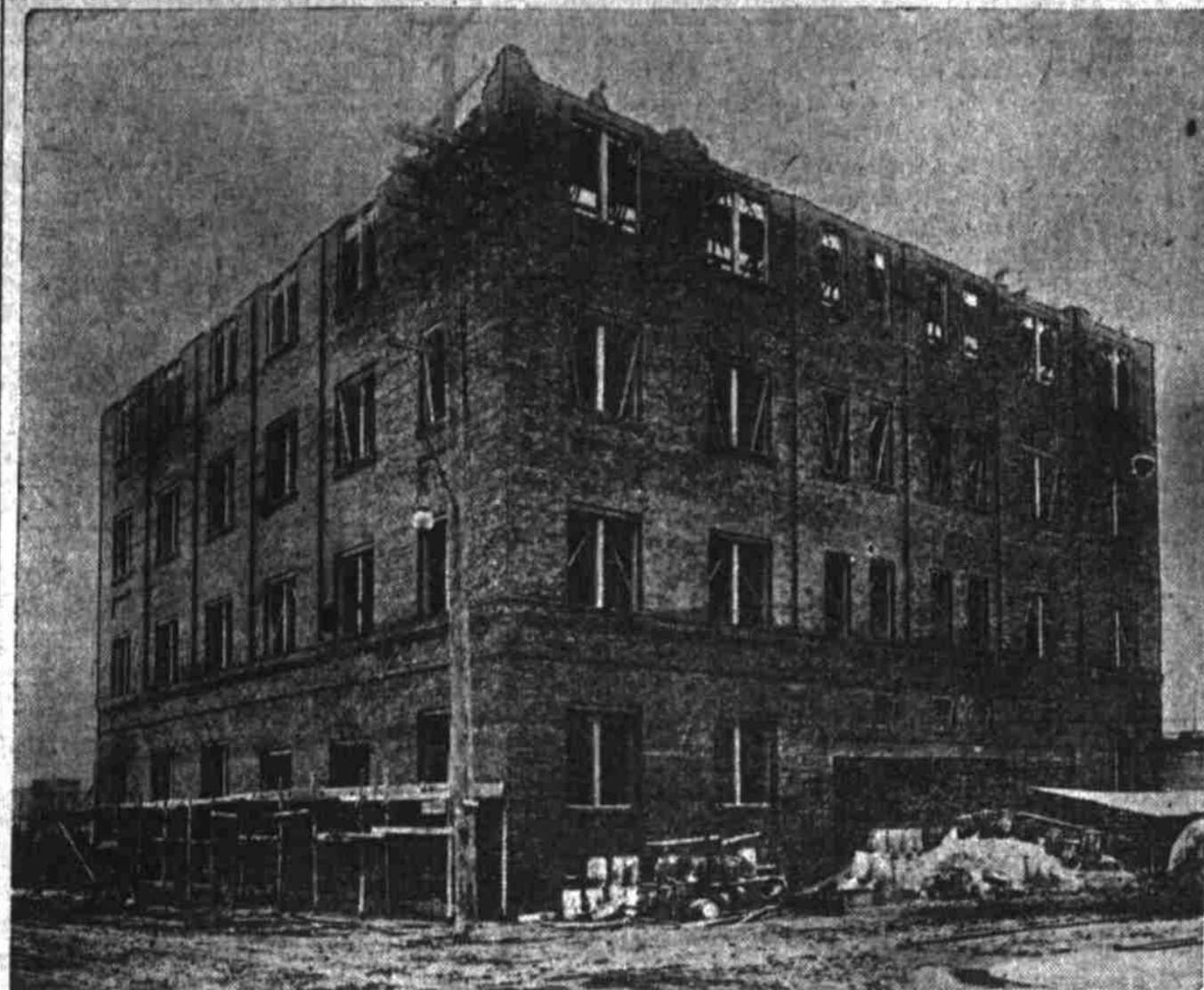
Birx Brothers' New Building at Twelfth and Glisan Streets.
