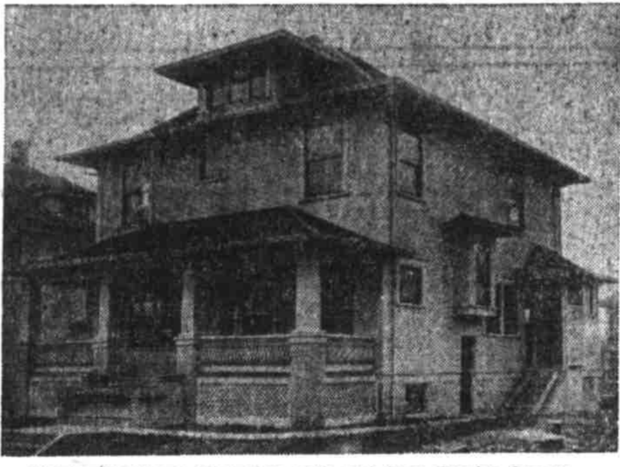
Ralston Residence, East Fourth and East Yamhill Streets.
