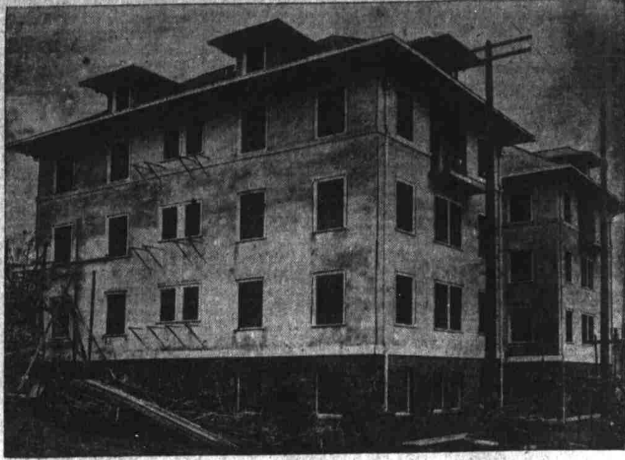
Spencer Apartments, King and Wayne Streets.
