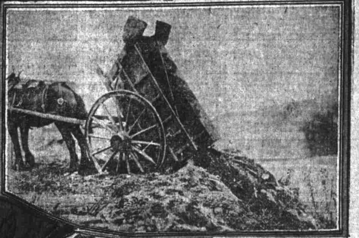
Contractors Dump Refuse into River
