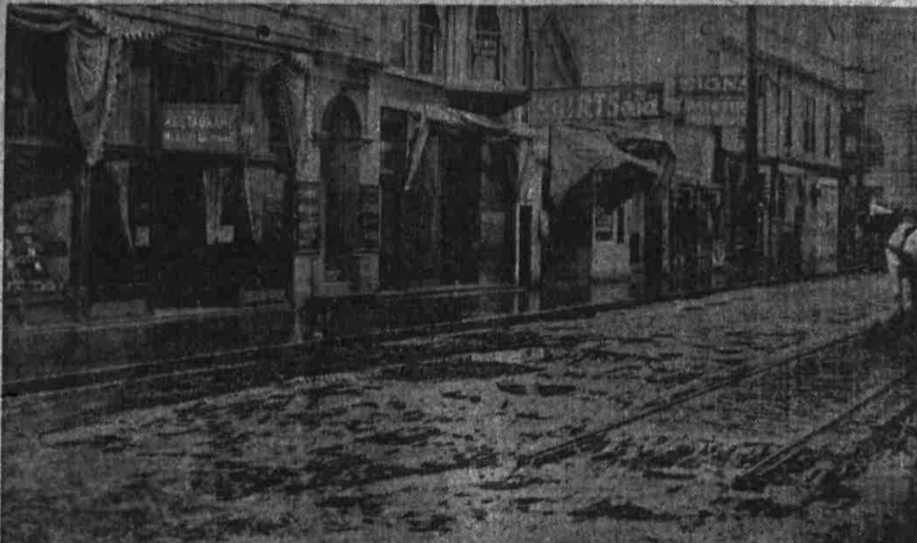
Terrible Condition of Stark Street Near the Corner of Fifth.
