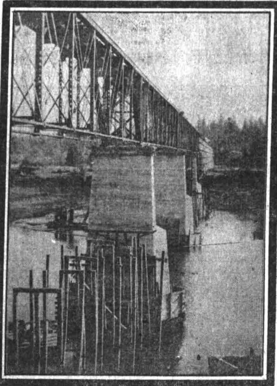
STEEL BRIDGE AT WILSONVILLE.
