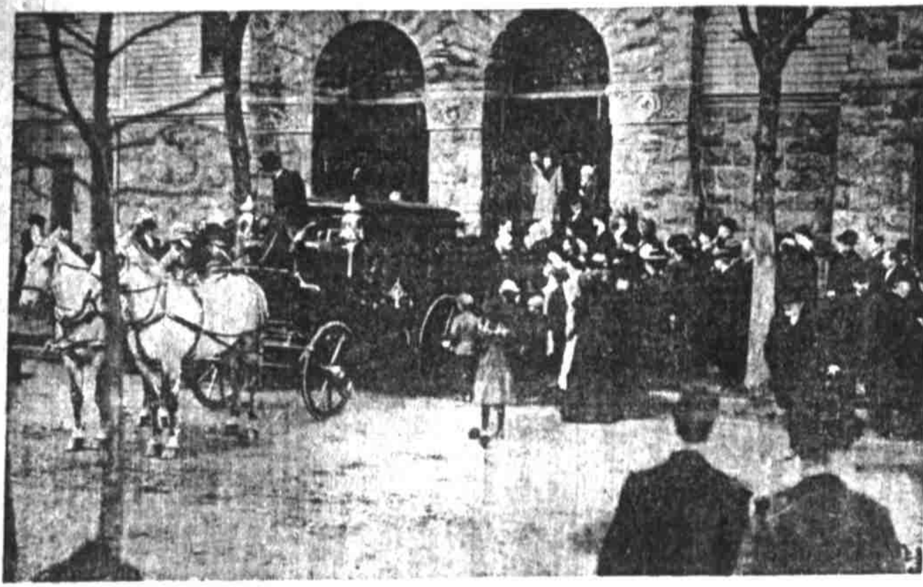
Scene in Front of Grace Church Yesterday Afternoon When the Remains of Judge A. L. Frazer Were Being Placed in the Hearse.
