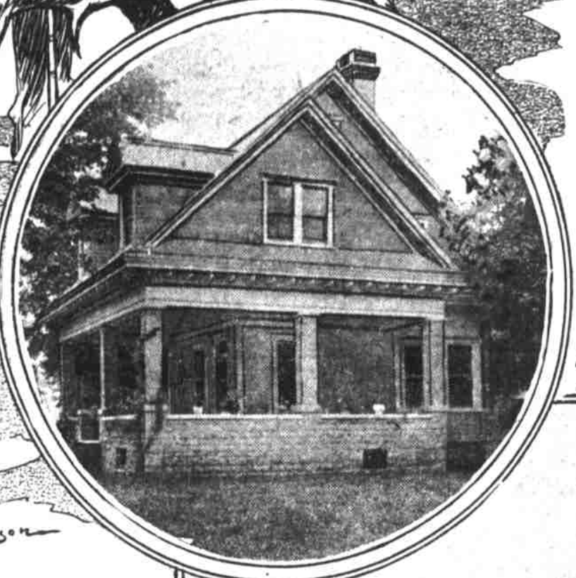
Cooper Office, Where all the Records are Kept.
