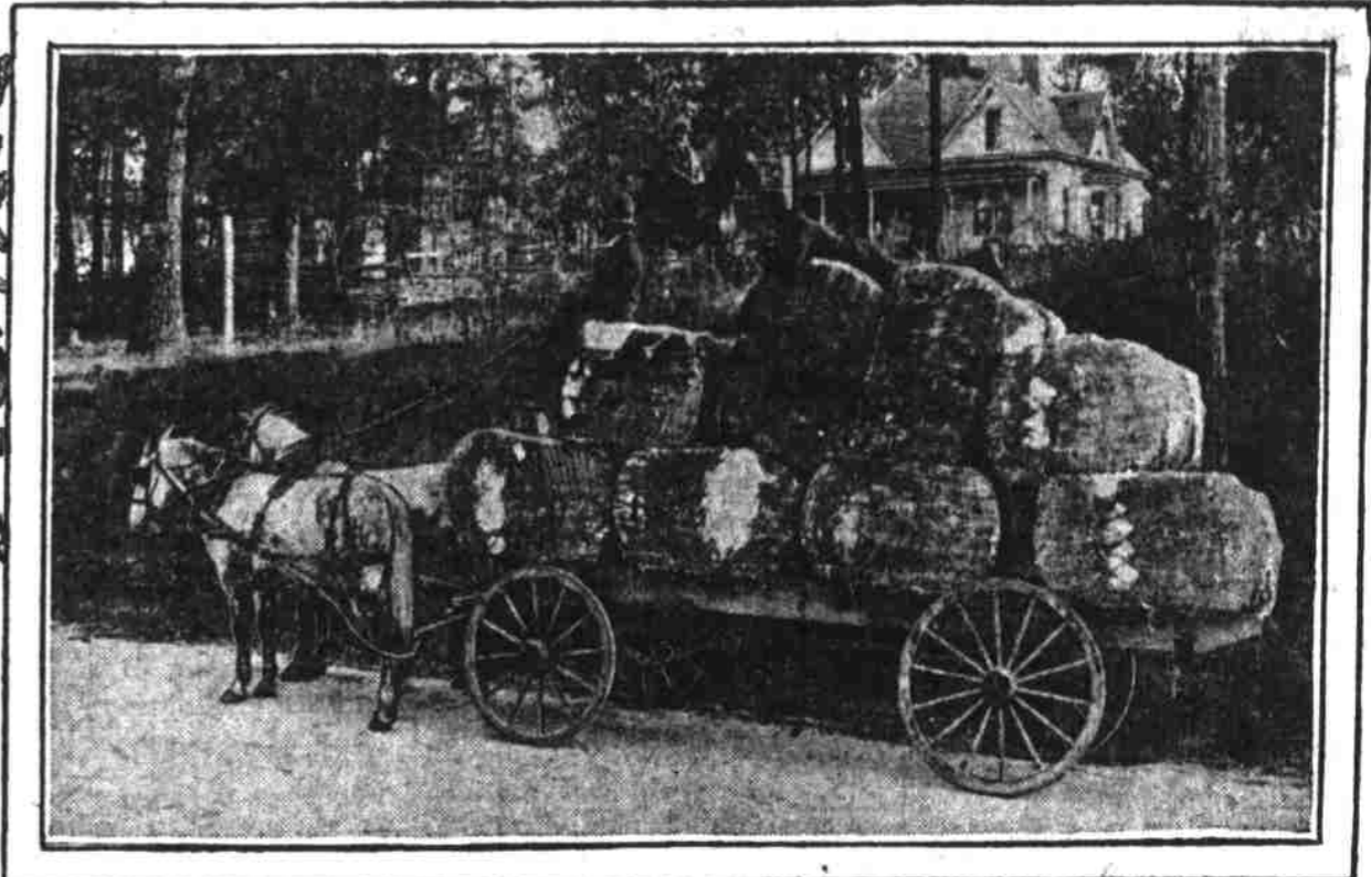
The Same Road, Improved, Permits Much Greater Load
