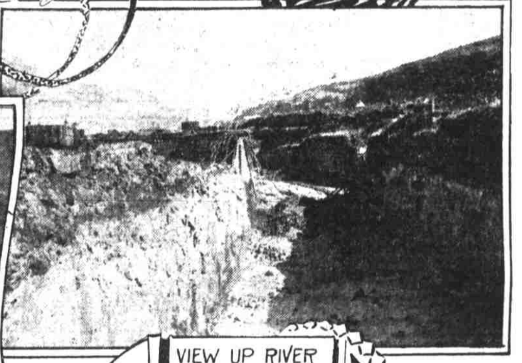
VIEW UP RIVER FROM SITE OF FIRST LOCK
