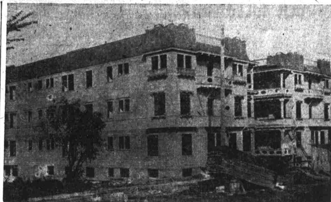
Irving Apartment House, Irving Street, Between Twenty-First and Twenty-Second Streets.
