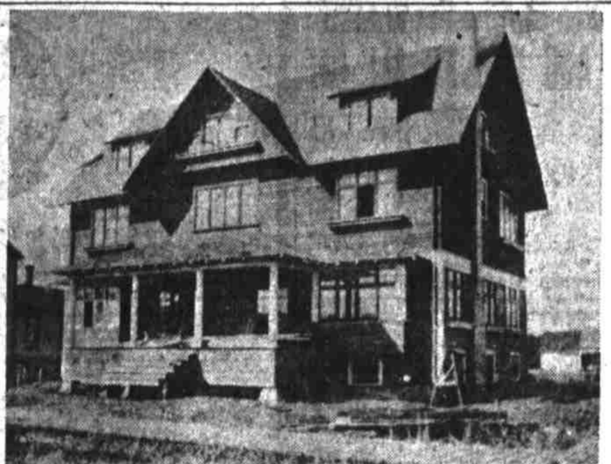
Tau Pi Sorority House, U. of O., Nearing Completion.
