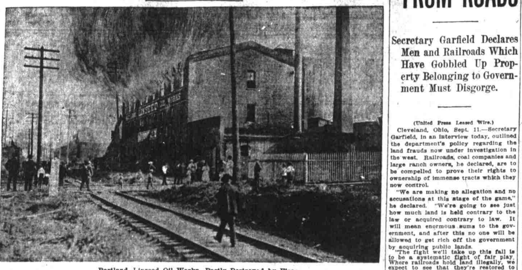
Portland Linseed Oil Works, Partly Destroyed by Fire.
