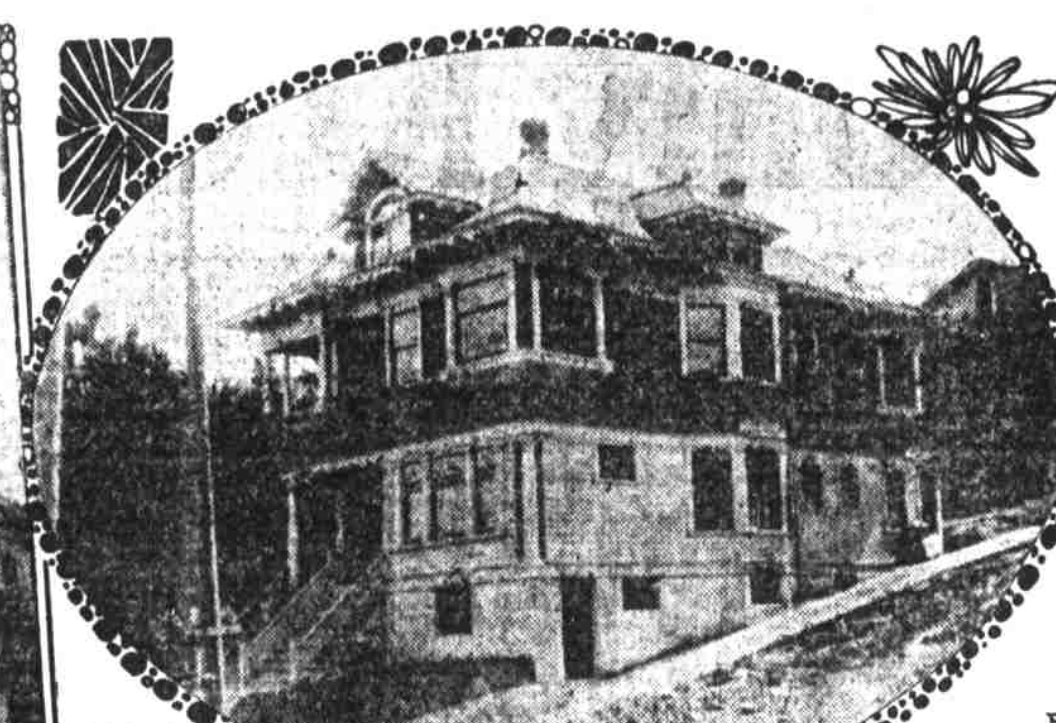
TYPE OF FLATS GOING UP AT 16TH AND MONTGOMERY STS.
