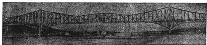
Spanning the St. Lawrence river at quebec, the huge steel bridge that gave way and dropped into the river below with such frightful loss of life, had the longest single span in the world. — Between the two anchor spans there was a channel span 1,800 feet long. It was total length of the structure was 3,300 feet, with a ship clear headway 150 feet above high tide. The height of the cantilever towers is 350 feet above high tide. The height of the cantilever towers is 350 feet above t
