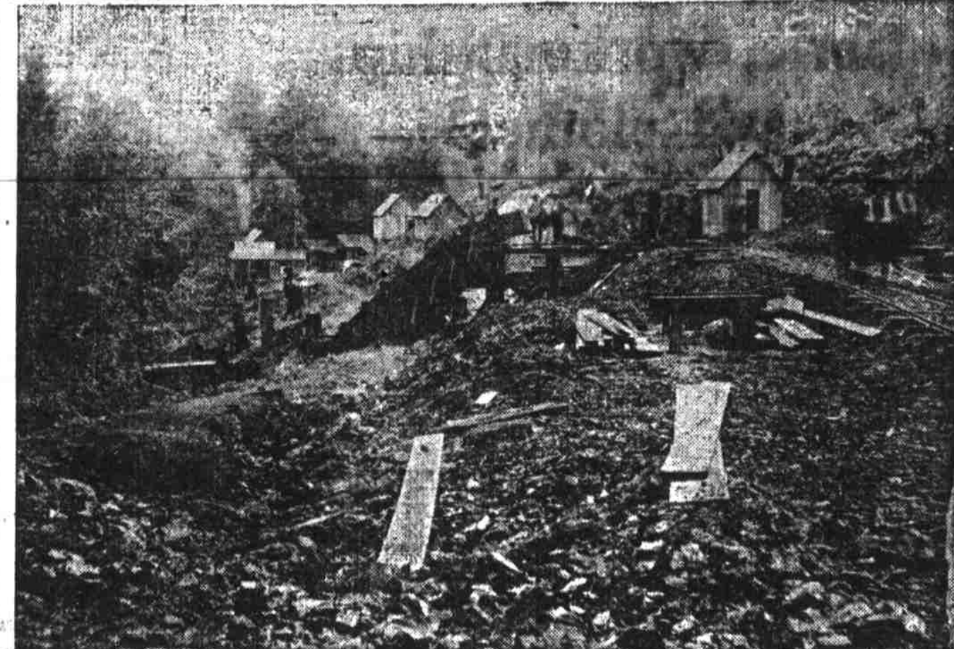
Quarters for Day and Night Shifts Are Being Rapidly Erected.
