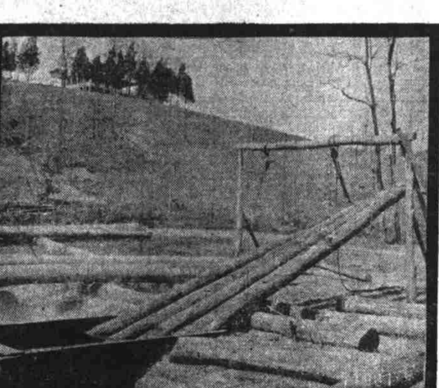
OPEN TANK TREATMENT OF POLES SHOWING BUTTS SUBMERGED IN CREOSOTE OIL.
