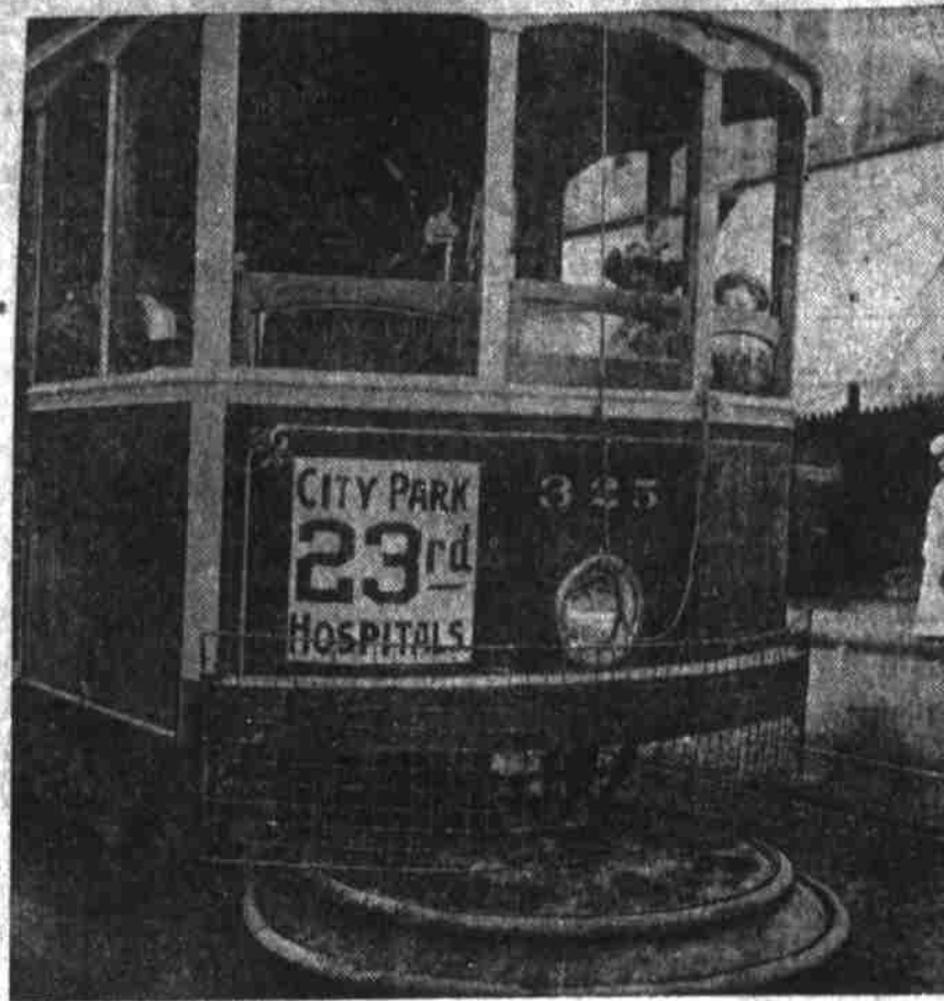
Unique Fender Invented by W. J. Haight for Portland Streetcars.
