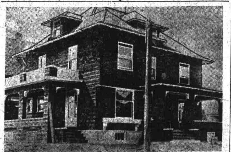
New Flats of F. F. Jancke at East Twelfth and Madison Streets.
