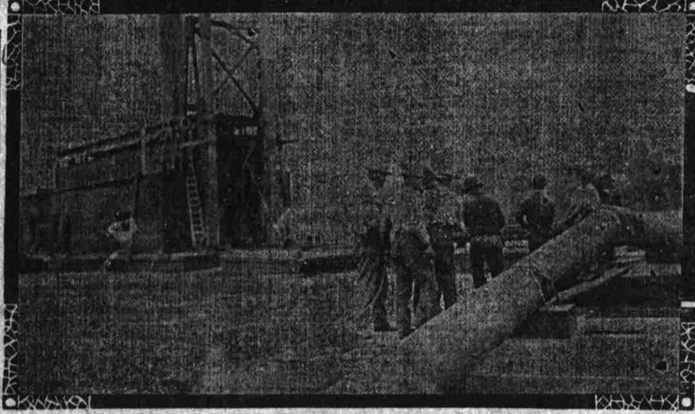
Big Dredge Starting on Fill for Packing Plant Site and Quarters of the Men at Work.
