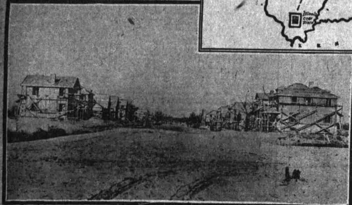
Building a city on the sand dunes.
