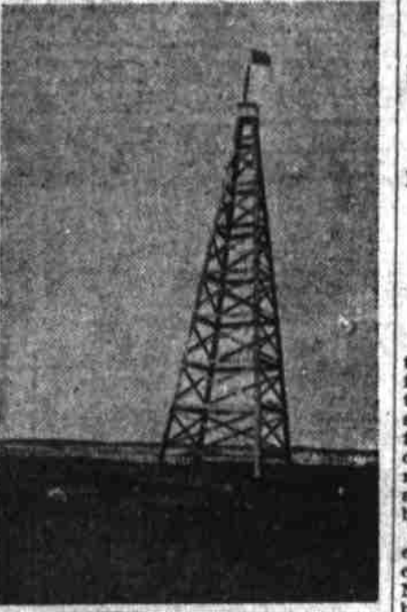
Seventy-Two-Foot Standard Derrick Built at Ontario, Oregon.
