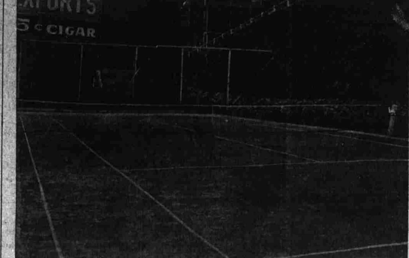
One of the New Asphalt Tennis Courts at the Multnomah Club.
