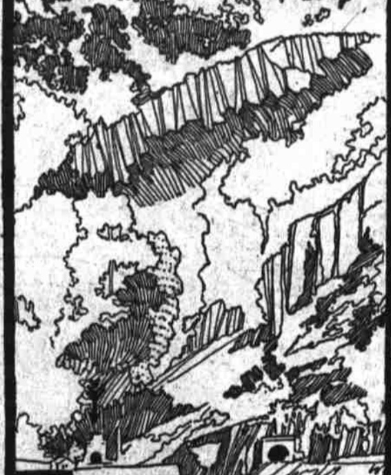
Where the Simplon Tunnel Boldly Plunges into the Alps
