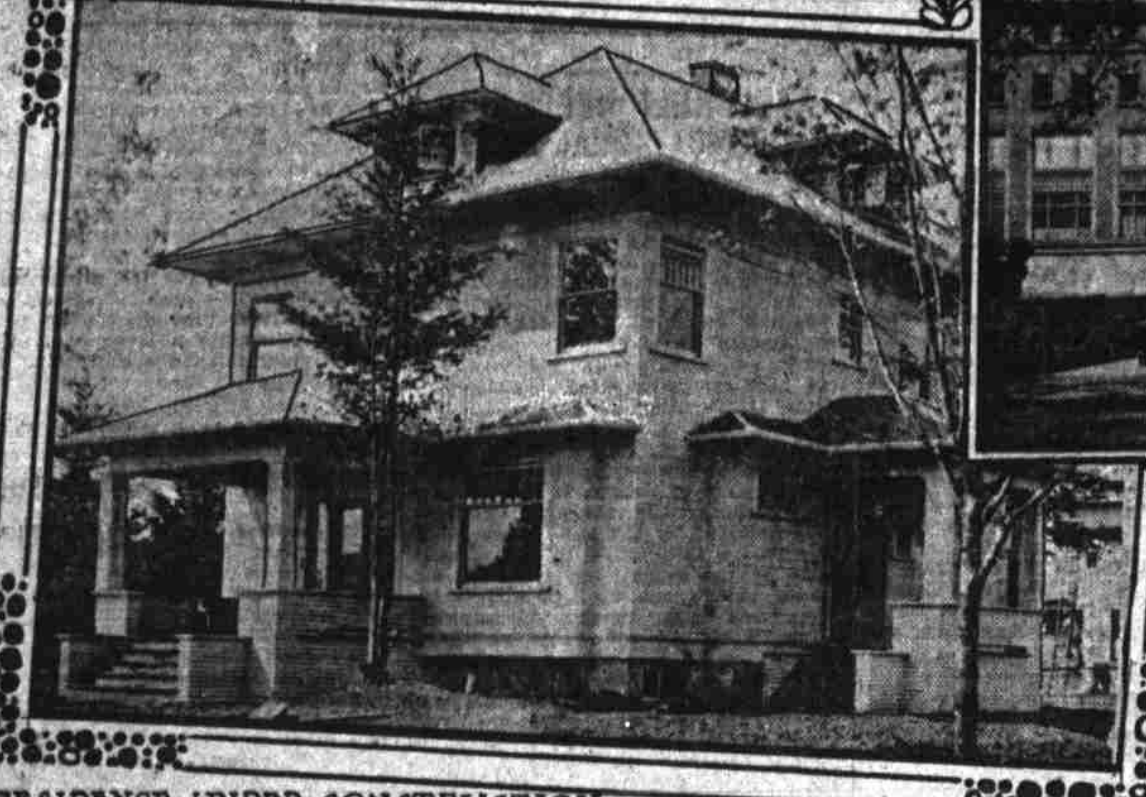
RESIDENCE UNDER CONSTRUCTION BY HERDMAN BROS. E. 22ND & WEIDLER.
