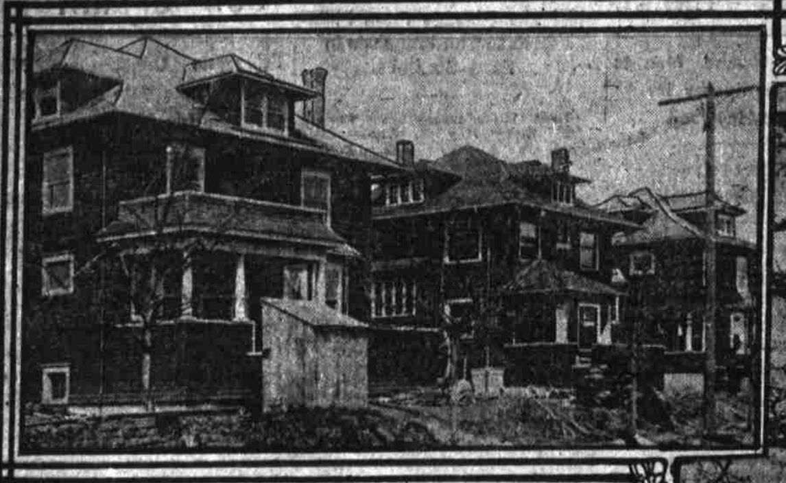
TYPE OF RESIDENCES UNDER CONSTRUCTION AT IRVINGTON
