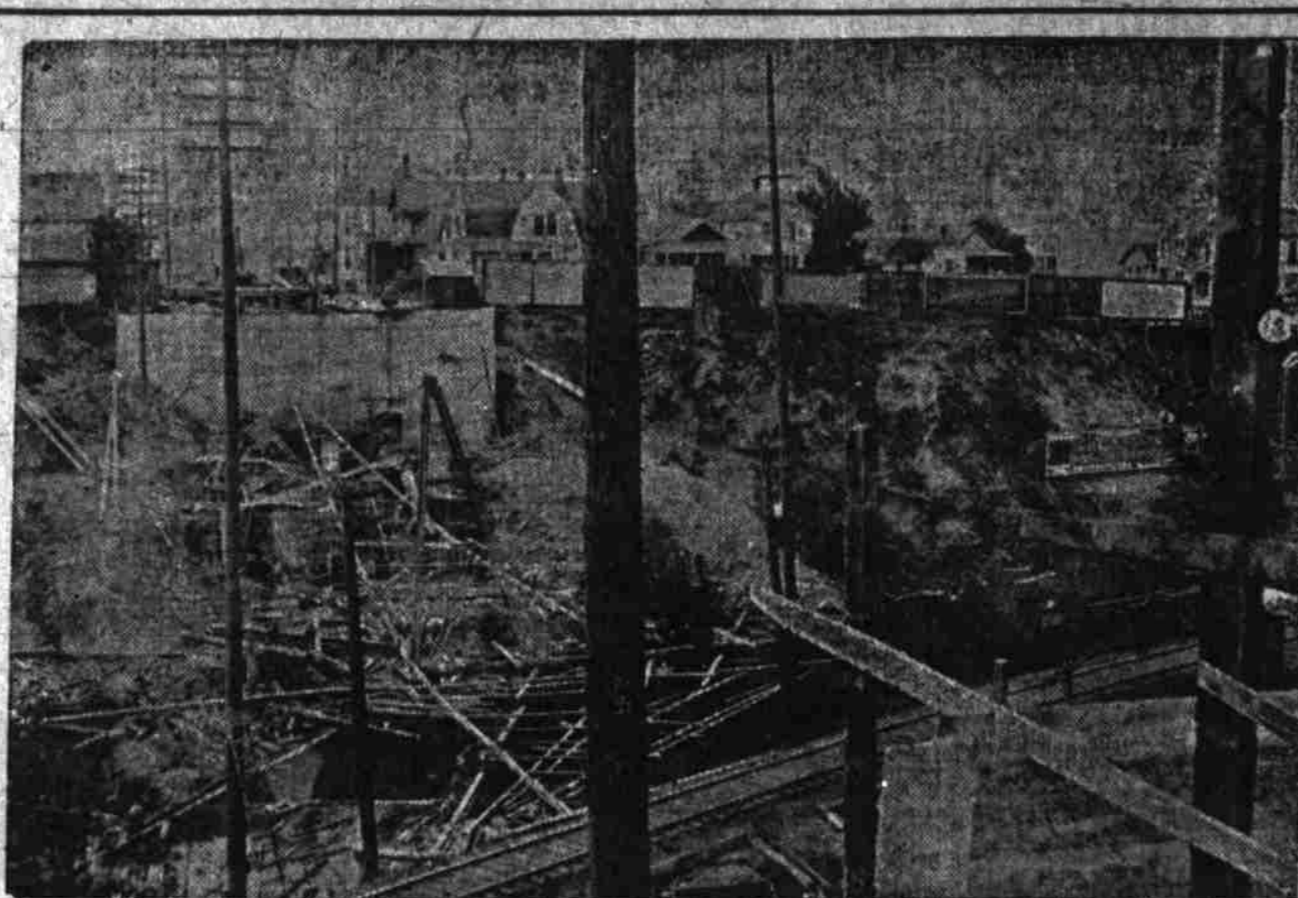
Concrete Abutments for Grand Avenue Bridge Over Sullivan's Gulch.
