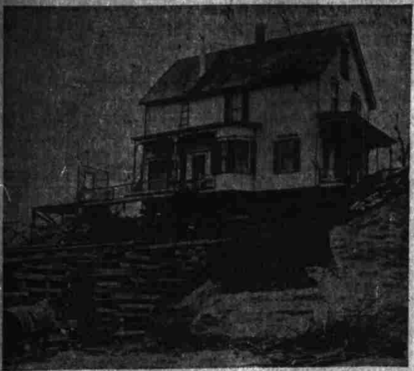
Moving Residence at Corner of Mississippi Avenue and Goldsmith Street.
