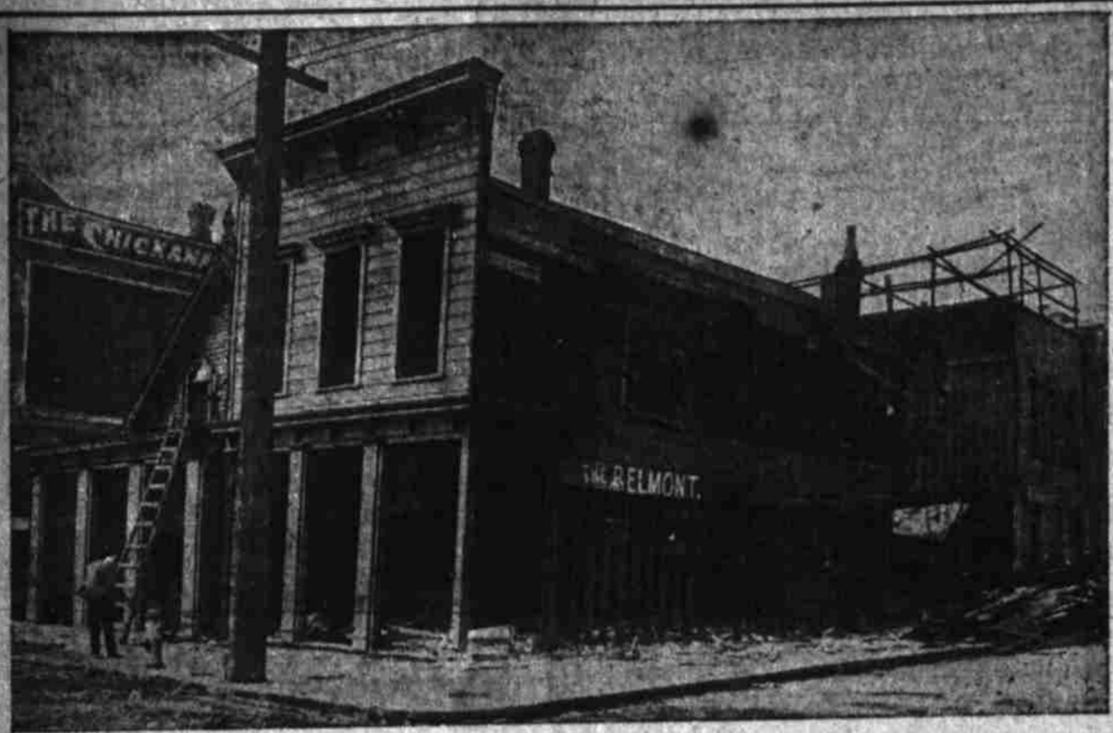
Shacks Torn Down at the Southwest Corner of Second and Salmon.
