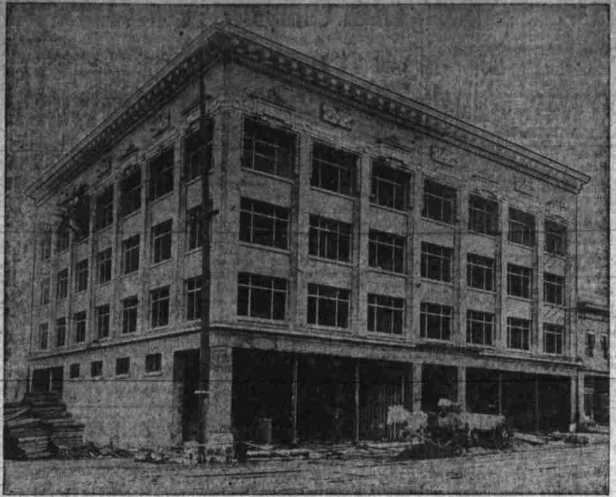
Jorgenson Building, Nearing Completion at Third and Main Streets.
