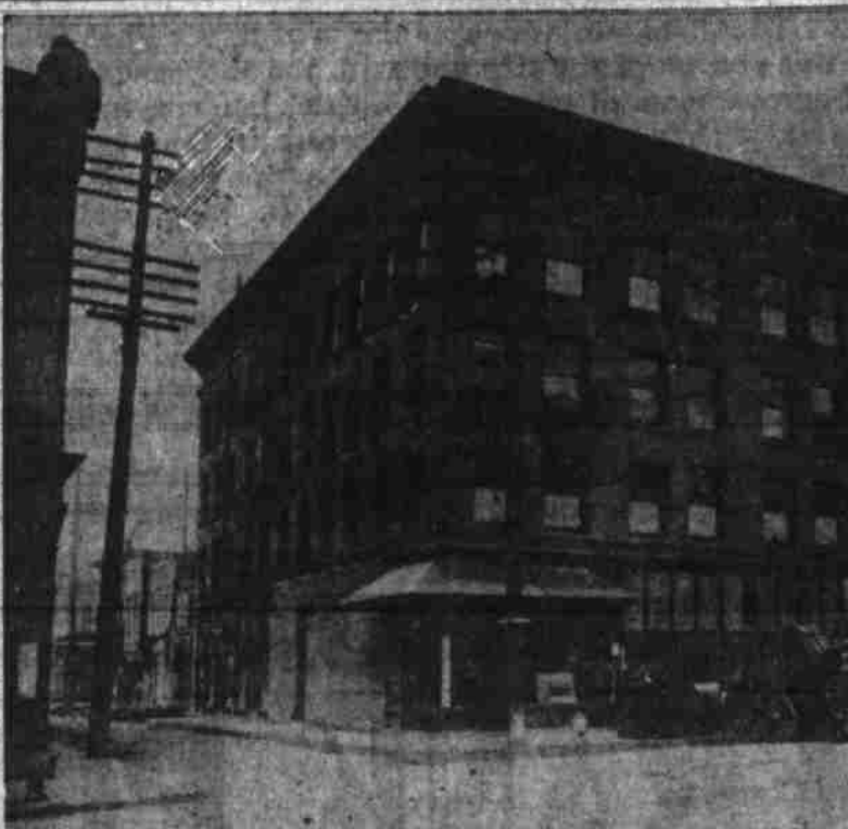
New Business Block, Built by J. F. Shea, at a Cost of $75,000, on the Northwest Corner of Second and Ankeny Streets.
