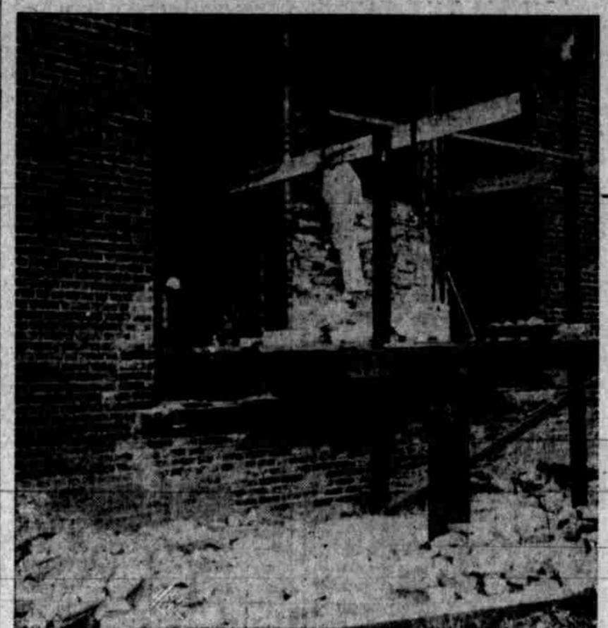
Where the Engine Poked Its Nose Through the Wall.
