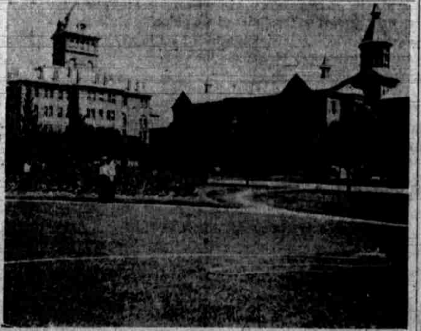
Agnew Asylum, Near San Jose, Which Collapsed, Killing More Than One Hundred Persons.
