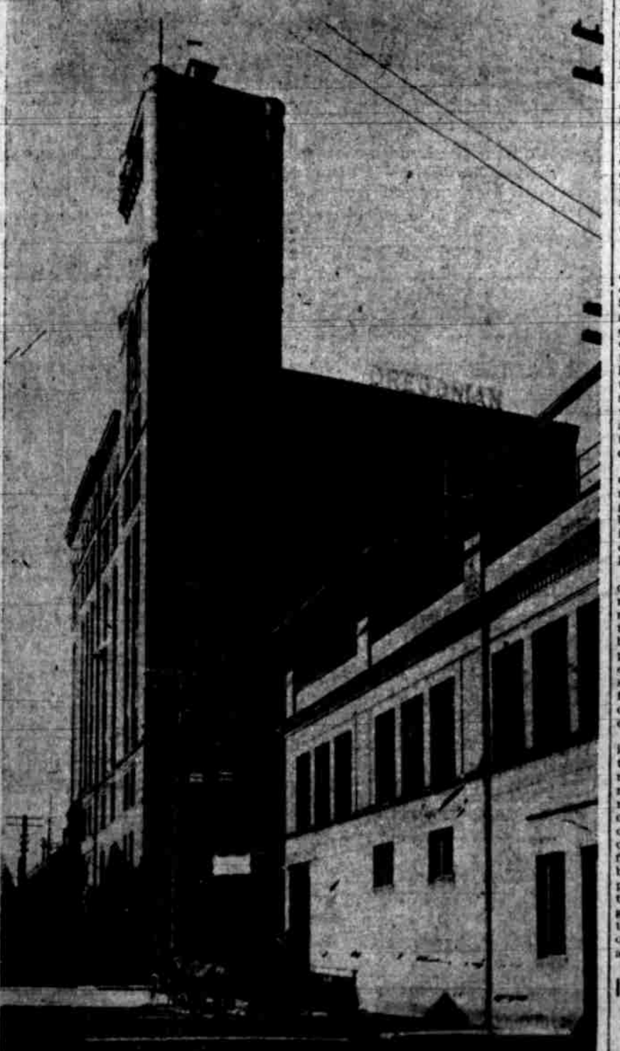
The Oregonian Building, One of the City's Conspicuous Examples of the Disregard of Laws Relating to Fire Escapes.
