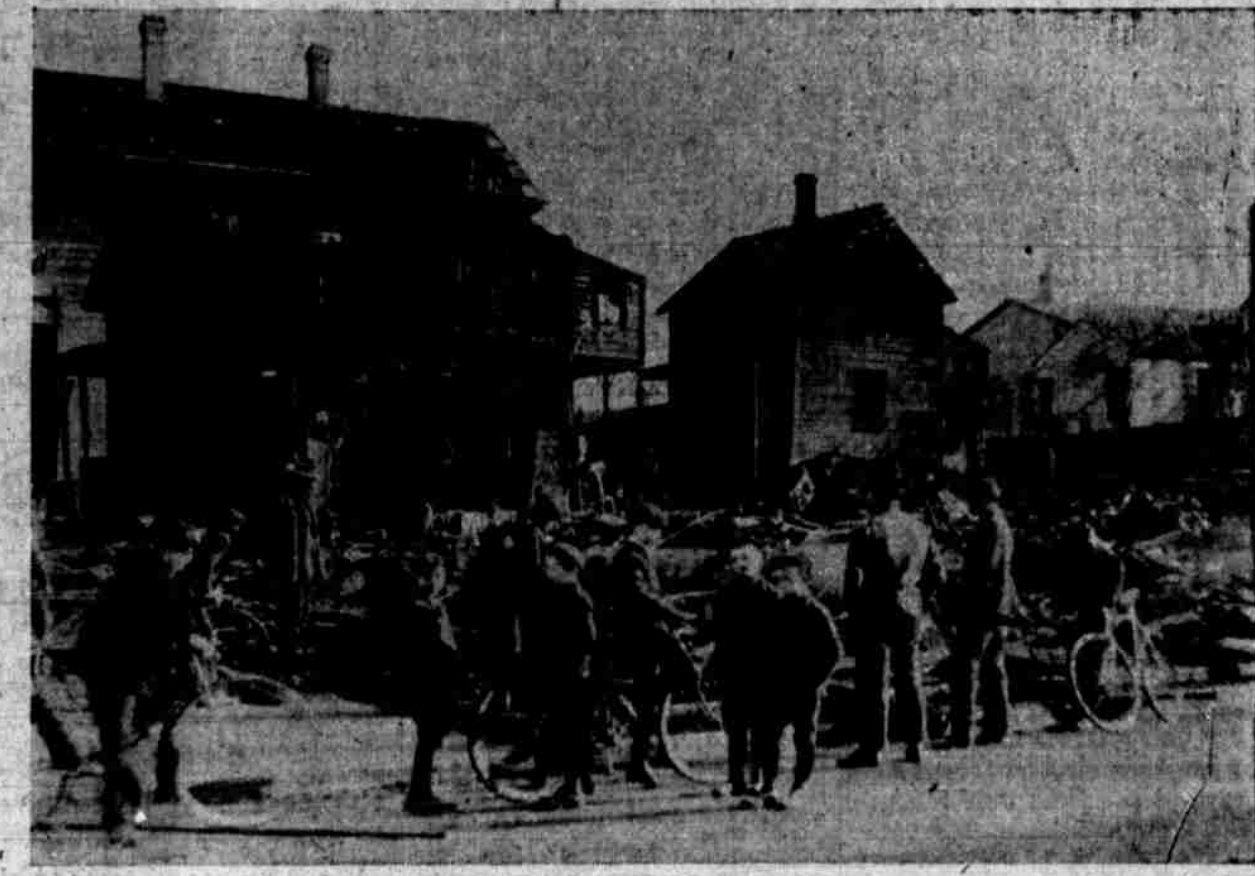
Shells of Buildings, Results of Last Night's Fire.
