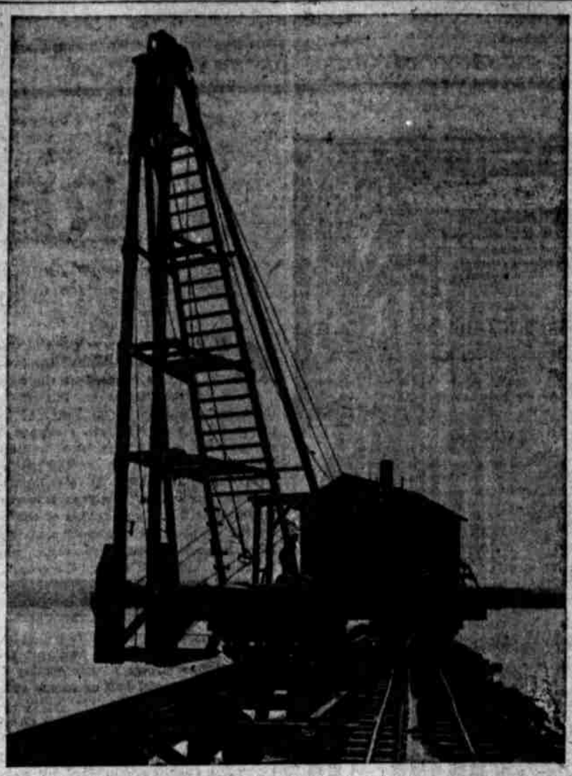
Driving Piles on the End of the Jetty.
